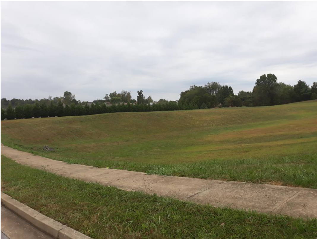
Wet weather conveyance on site (View from Willow Springs Dr)
